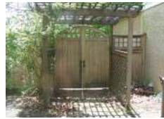
Pergola & Gate Before
